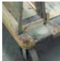
Wood—splinters and rot
